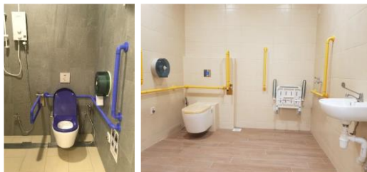
Figure 5 – Examples of toilets (colour contrast between toilet seat and cover, grab bars at water closet and shower area)
